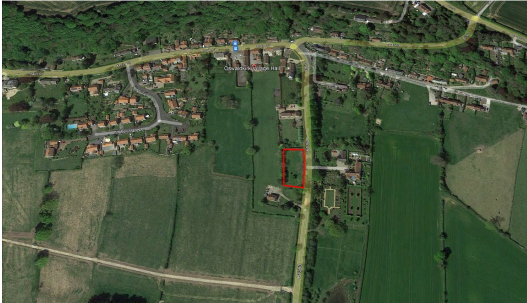
Figure 1.1 Site Location and Context.
